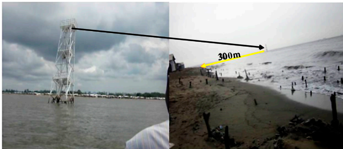
Figure 12. Illustration of the rising waters, with the immersion of the communication relay antenna in the sea, installed off the mainland of Cap Cameroun around 1993 (adapted from the study of Tchindjang et al. [38] based on vulnerability and adaptation of Cap Cameroun populations to natural risks).
