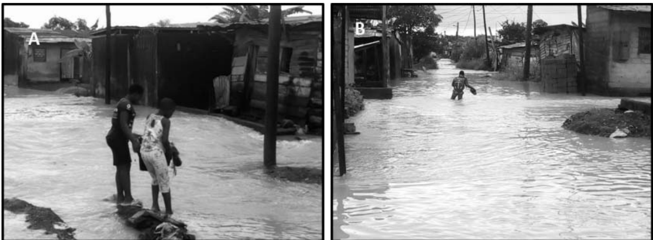
Figure 9. Some anthropogenic activities that promote flooding in the Tongo Bassa watershed in Douala: (A) dumping of household waste into the waters during the flood of 21 August 2020; and (B) construction in low areas close to watercourses.
